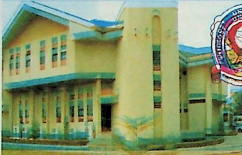
James McKeown Auditorium James McKeown Auditorium Air-conditioned Conference Hall
